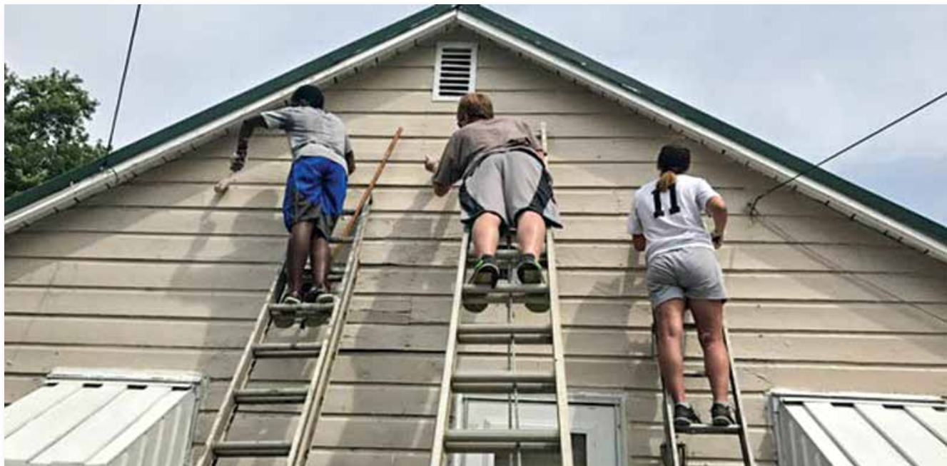
During the day, young Christians participating in the Mid-Ohio Valley Work Camp paint the home of Elizabeth Carro.
