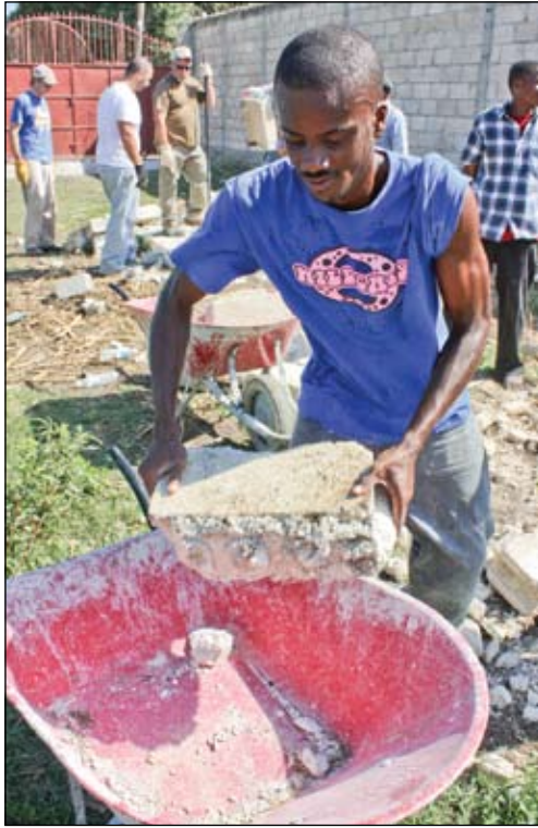
David and other residents of Son Light move broken concrete with help from U.S. volunteers.
