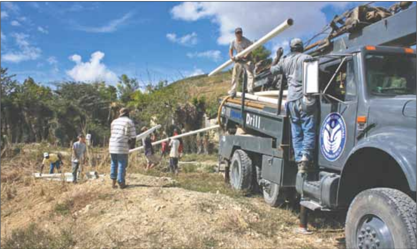
Workers representing Healing Hands International unload tubing at the site of a new water well in a community near Port-au-Prince.
