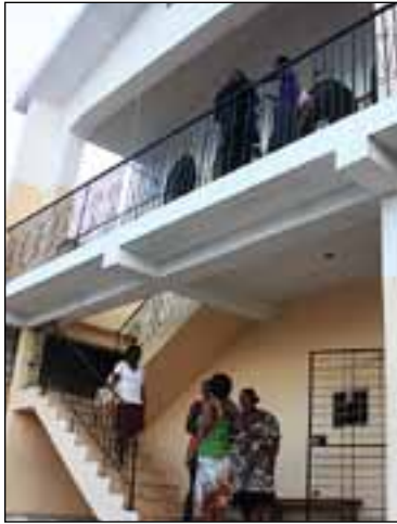
PHOTOS BY ERIK TRYGGESTAD The refurbished meeting place of the Bolosse Church of Christ.
