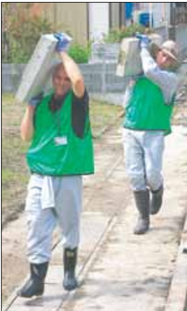
Larry Musick and Jonathan Straker replace pavers on a sewer.
