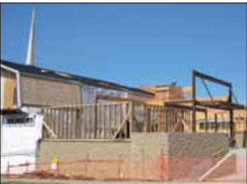
Construction proceeds on an expansion project at the Holgate Church of Christ.
