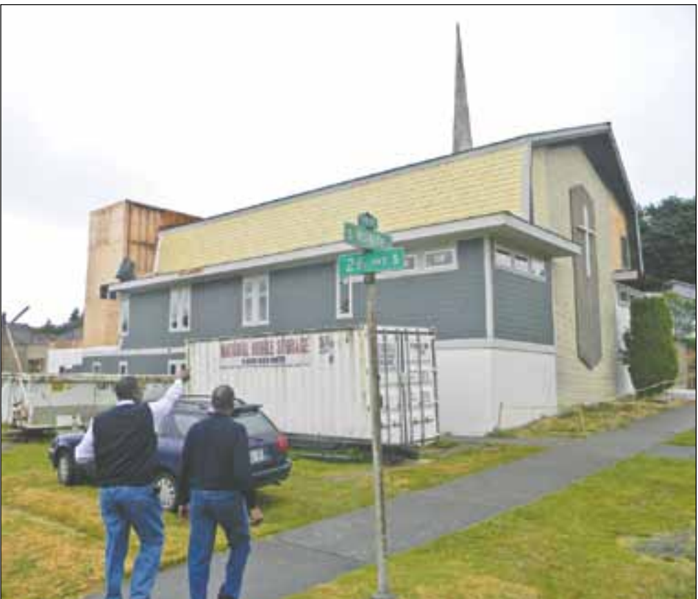
Minister James A. Maxwell and church financial secretary Robert Stowers check on the status of construction. The 11,000-square-foot building is being expanded to about 28,000 square feet.
