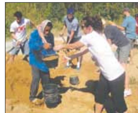
The mission team works side by side with Thais to set a church building’s foundation.
