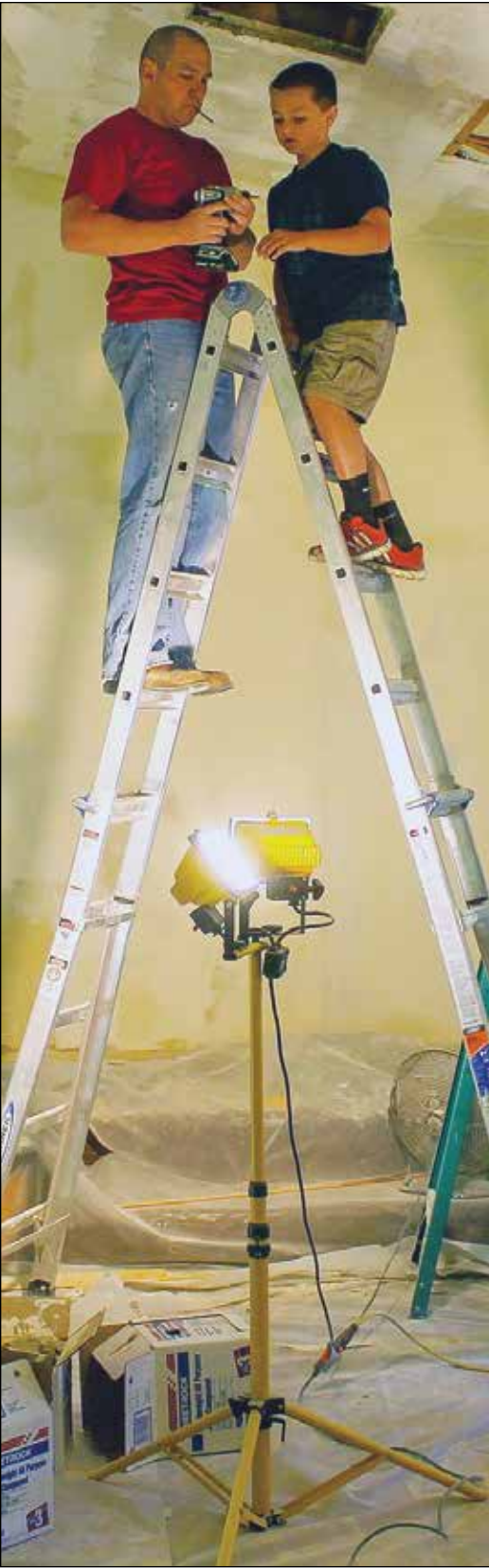
Rick Owens and his son Carter Owens, 9, work on a ceiling project at the Logan Church of Christ.
