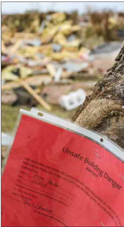
A sign on a tree next to the Pattersons' residence warns of the unsafe conditions after the storm. BOBBY ROSS JR.
