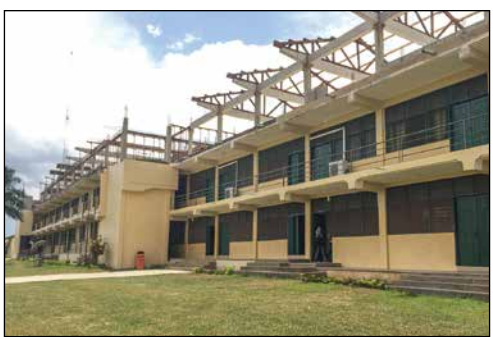
A third story of classrooms is under construction at Heritage Christian College in Accra, Ghana.
